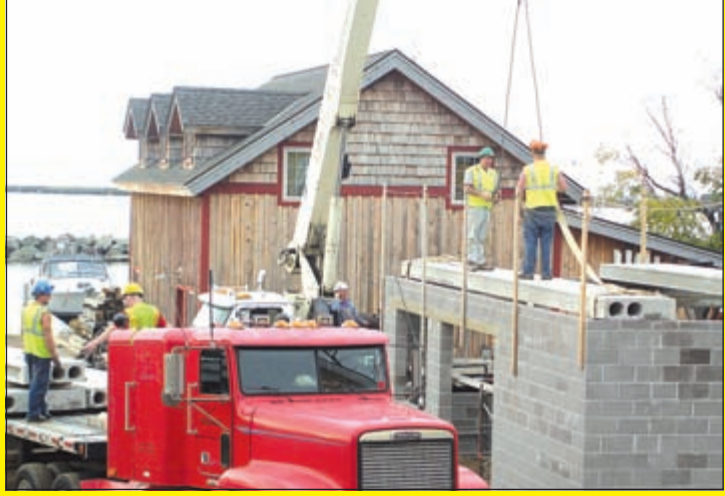
Erecting new building at North House Folk School 2008
