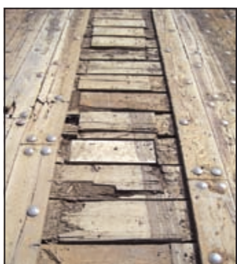
Photos courtesy of Cook County Highway Department The 50-year-old bridge at the end of the Arrowhead Trail may have reached the end of its lifespan. Left: The bridge's vertical timber pilings are starting to rot. Above: Car tires could be damaged or possibly drop through the bridge planks.
