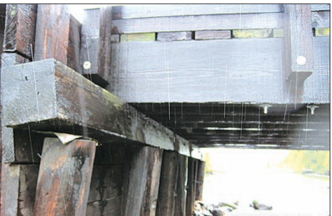
Photos courtesy of Cook County Highway Department The 50-year-old bridge at the end of the Arrowhead Trail may have reached the end of its lifespan. Left: The bridge's vertical timber pilings are starting to rot. Above: Car tires could be damaged or possibly drop through the bridge planks.
